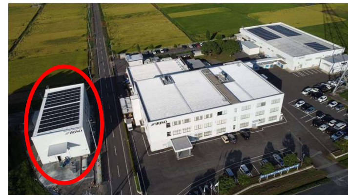
Ibaraki Plant New Building
